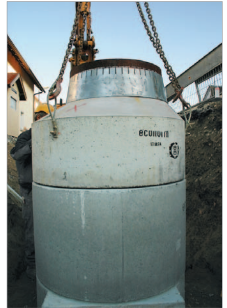
A manhole socket in position. Rapid installation without mortar using the connector system
